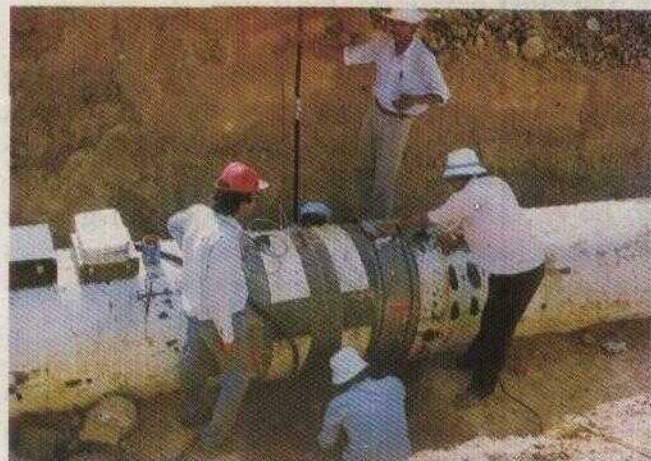
II. 10. Lowering of HBJ Gas Pipeline
