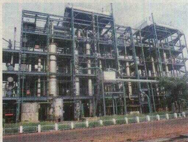
V.A.1 A View of Butanol Plant
