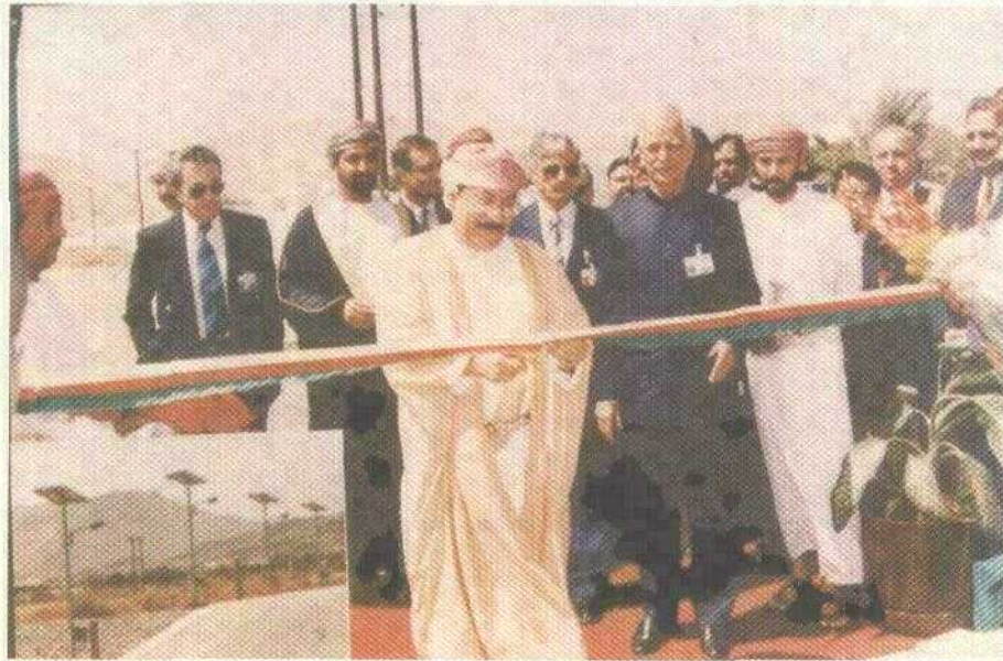
VIII.B.1 CEL's SPV Street Lights installed near Muscat in Oman (shown in inset) being inaugurated
