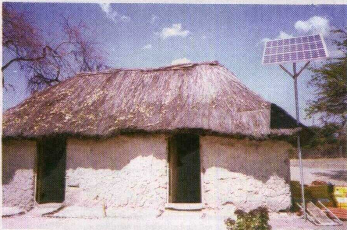
VIII.B.4 SPV Powered Domestic Lighting Systems by CEL in a village Spitzkoppe in Namibia
