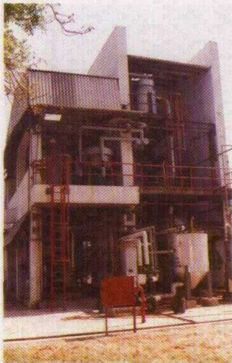
III.A.2 Per-acetic acid and Epoxidation of Alpha-Pinene plant
