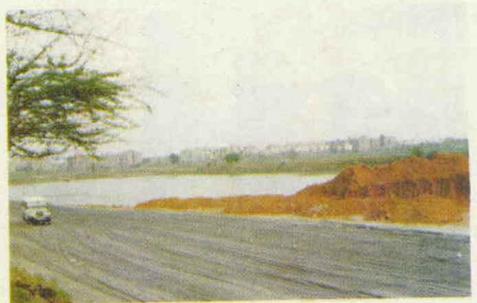
II.8 Flyash for highway embankment construction
