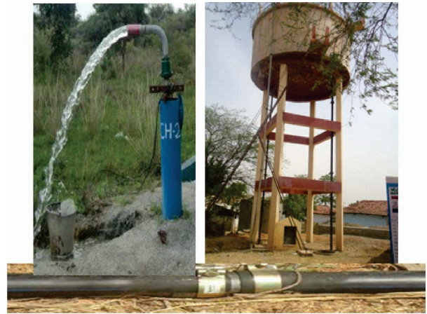
Water coming from bore-well and being carried to over-head tank of near by villages
