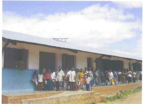
SPV System for a School in Mozambique
