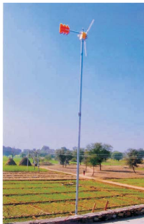
Fig. 3: Small PV-Wind Hybrid Power Plant for Rural Application
