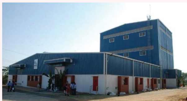
Side view of Palletization plant at NRPL site
