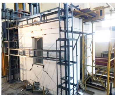
Damage pattern for retrofitted confined masonry building subjected to lateral cyclic load
