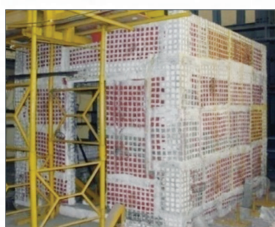
Plastering and curing
