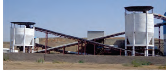
Overview of Lignite Beneficiation plant designed, erected, installed and commissioned by Ardee
