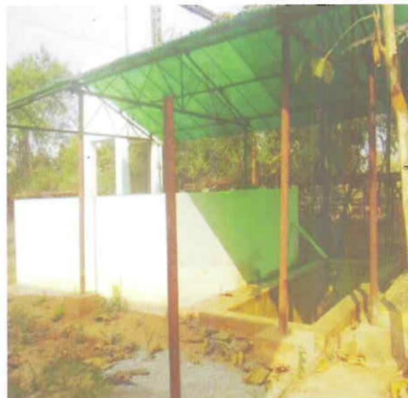
Ten ton bioleaching plant for nickel ore at IMMT
