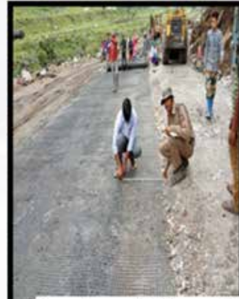
Laying of Geogrid on Subgrade
